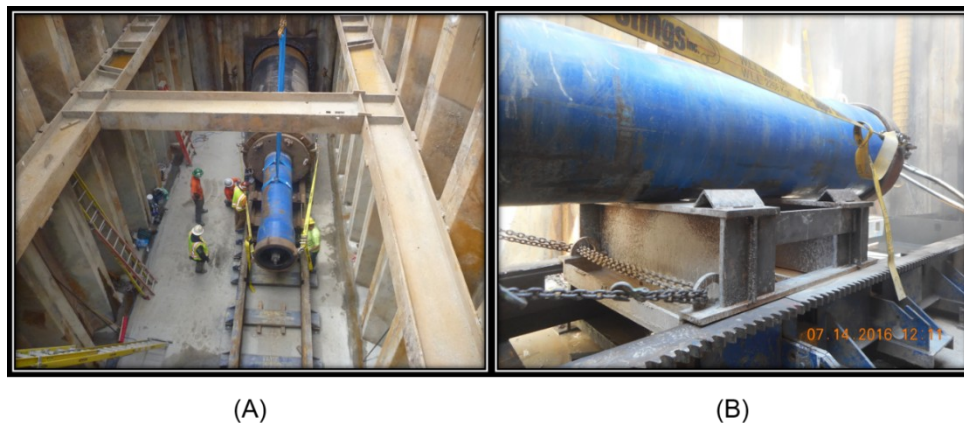
Figure 7 (A) Grundoram Taurus pneumatic hammer. (B) Hammer Sled to hold hammer to design grade.
