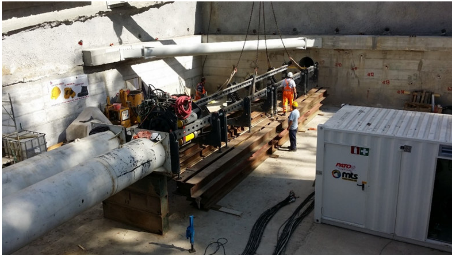
Fig. 18 jacking frame and control cabin
