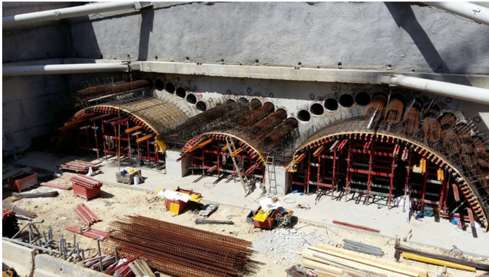
Fig. 22 – steel reinforcement cages
