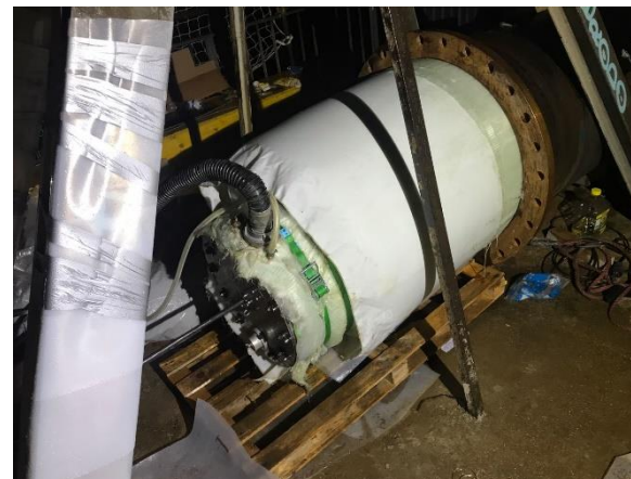
Liner pull-in and UV-curing
