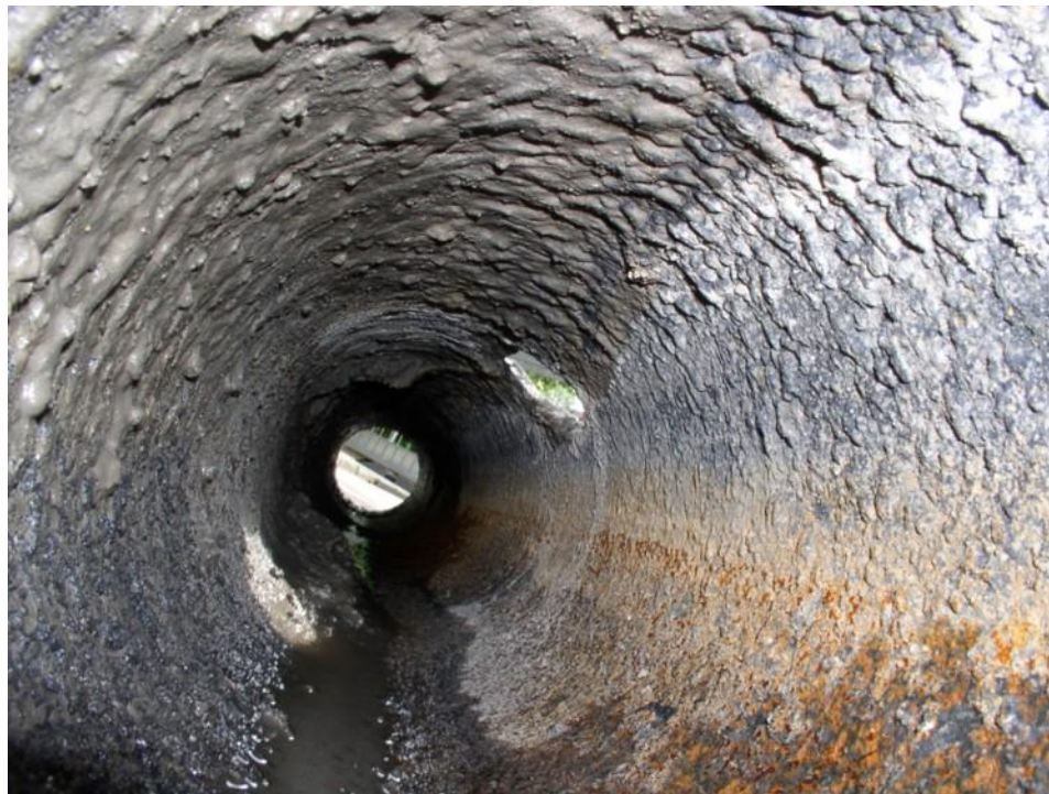
Inner corrosion
