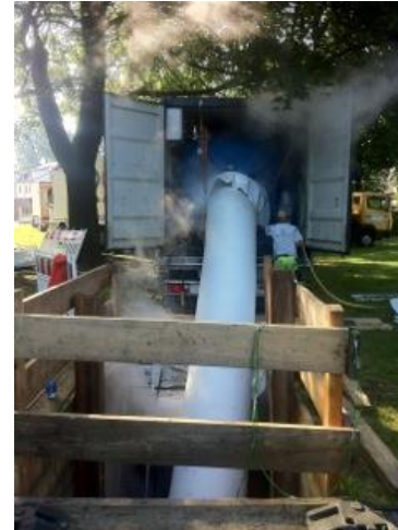
Liner inversion and steam curing
