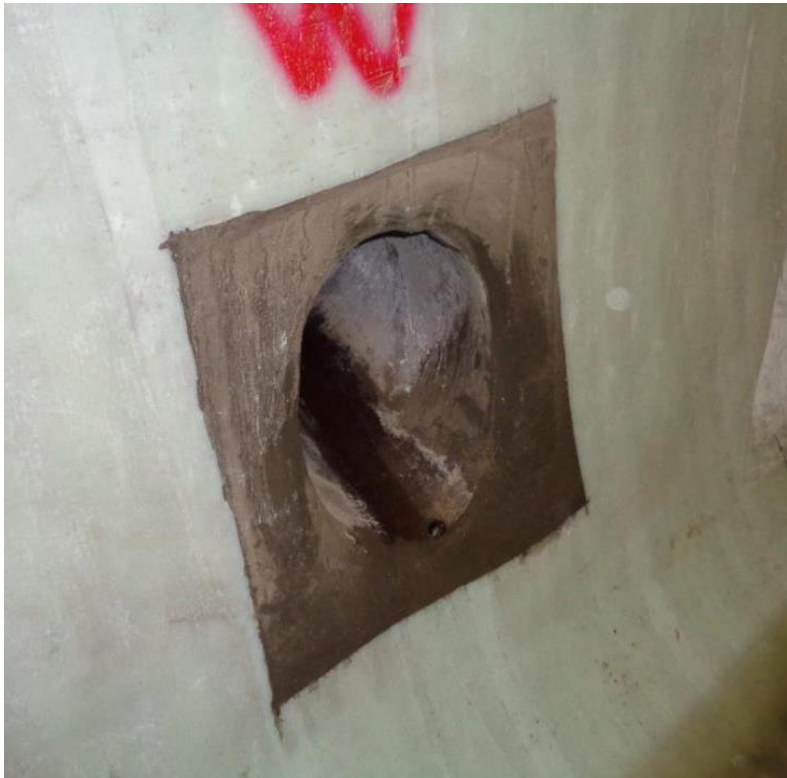
finishing and sealing of the connections
