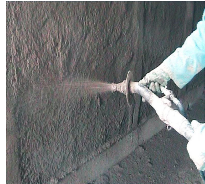
mortar spraying 2 times
