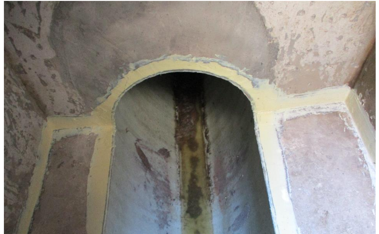
finishing and sealing of the liner
