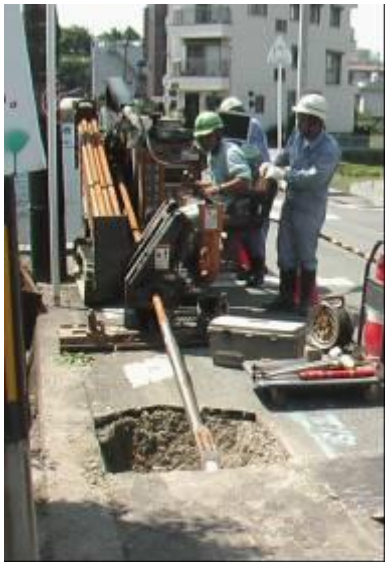
(b) Controlling the boring machine (c) Tip of the head with small antenna
