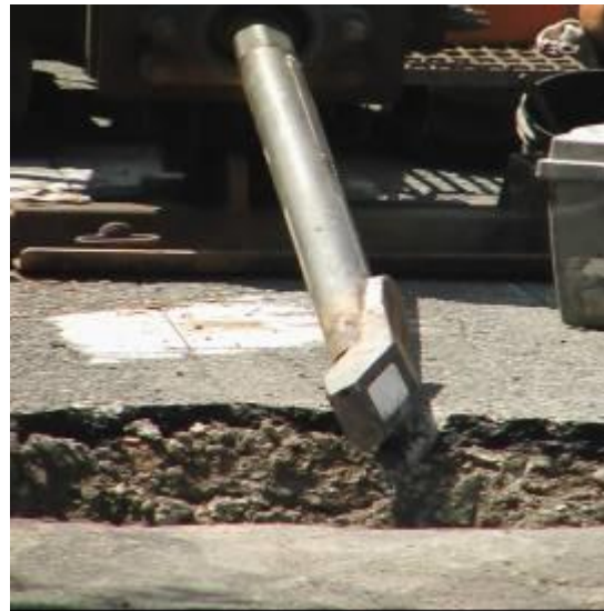
(b) Controlling the boring machine (c) Tip of the head with small antenna
