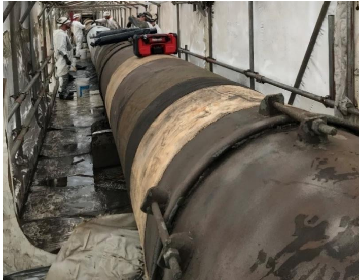
Step 1: Surface Preparation
