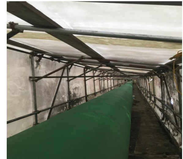
Step 3: Finish System applied
