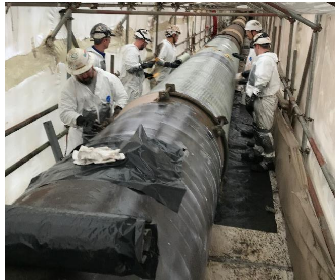
Step 2: Installation of GFRP/CFRP System
