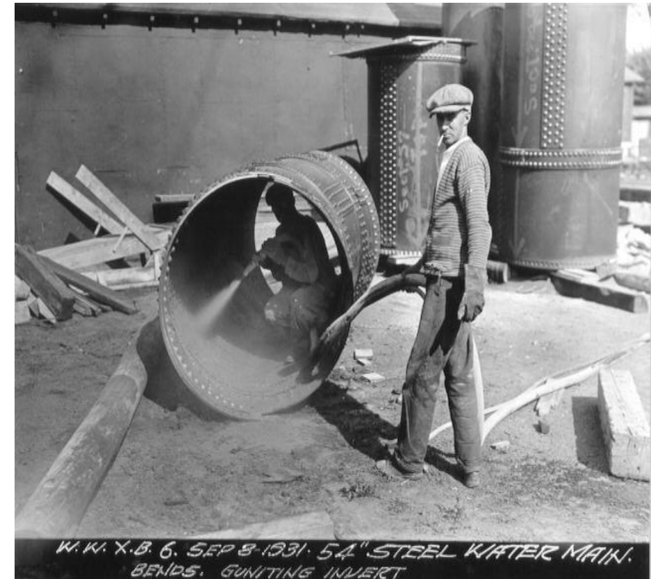
1200mm Riveted Steel Pipe using a 1350mm steel casing
