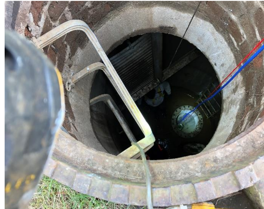
Installation and access point for 2100mm CCTV
