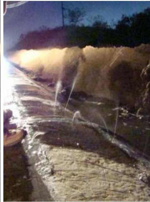
Leaks continued after cracks were filled
