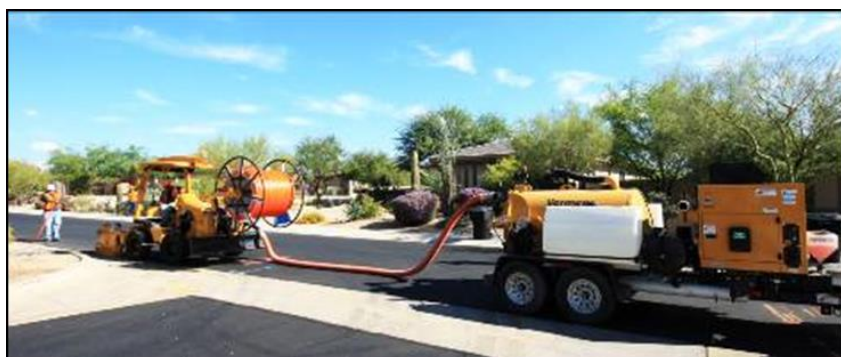
Micro-Trenching with Vacuum Excavation
