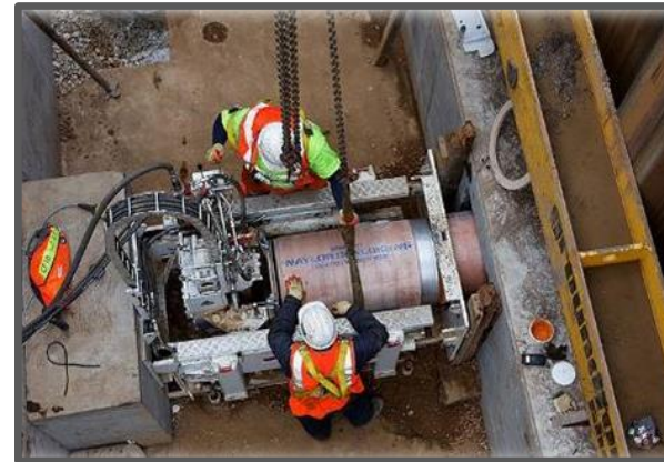
Auger Boring / Pipe Jacking
