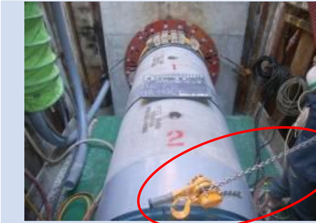
Figure 8. Safety measures taken at the start shaft
