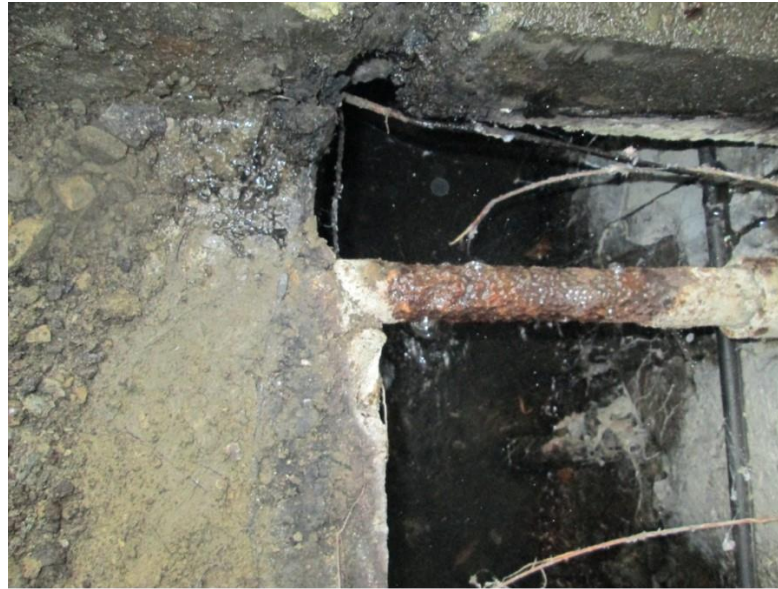
Corroded pipelines
