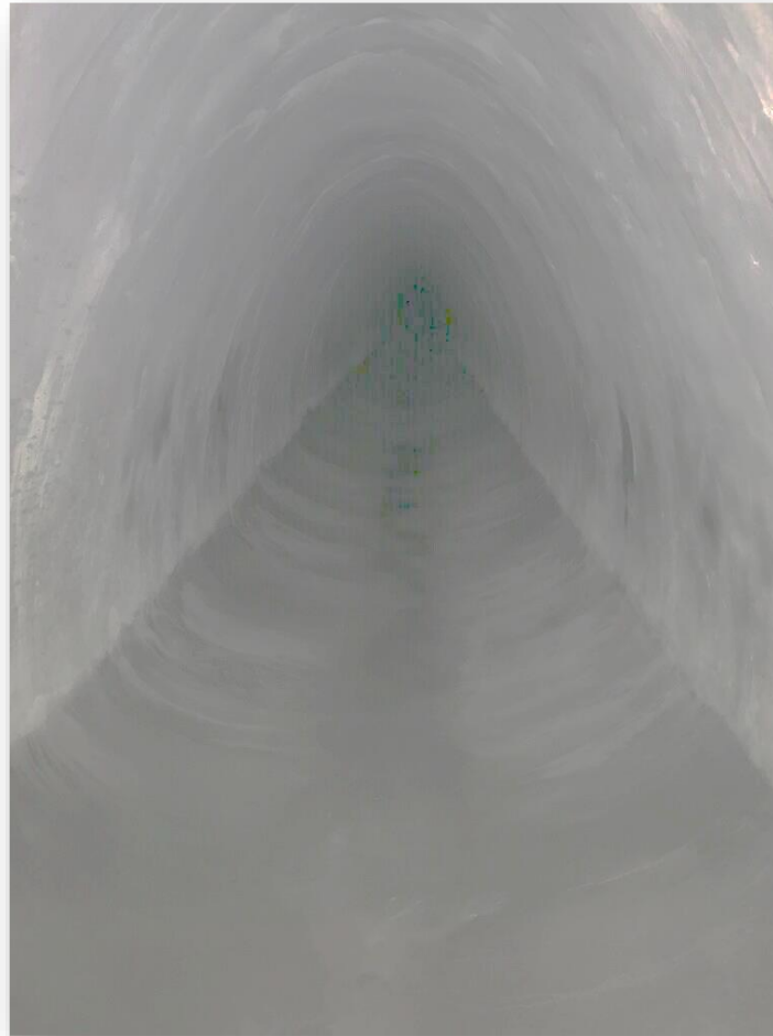
Pipe Structural Lining Completed
