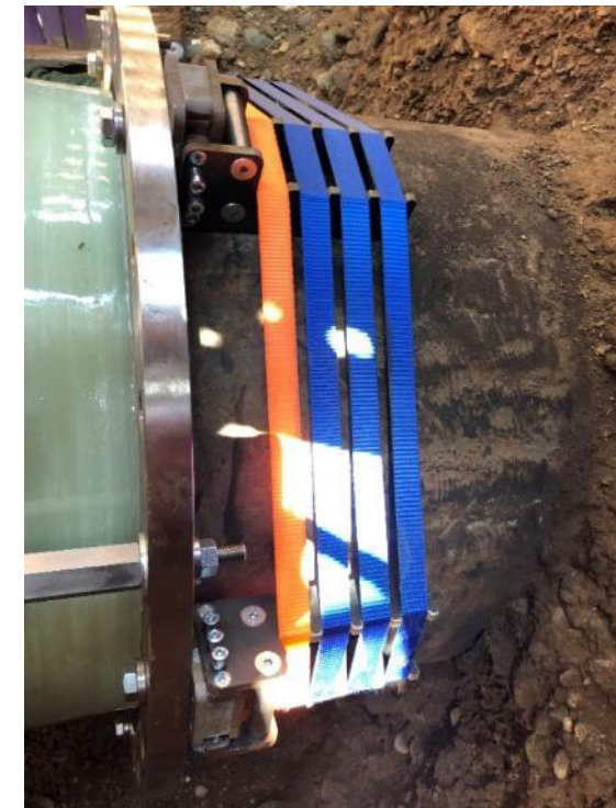
Fixation at host pipe
