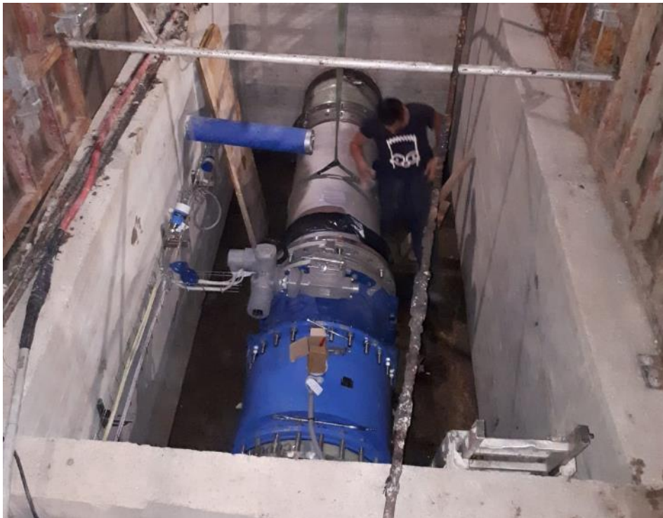
Connection works in a service chamber
