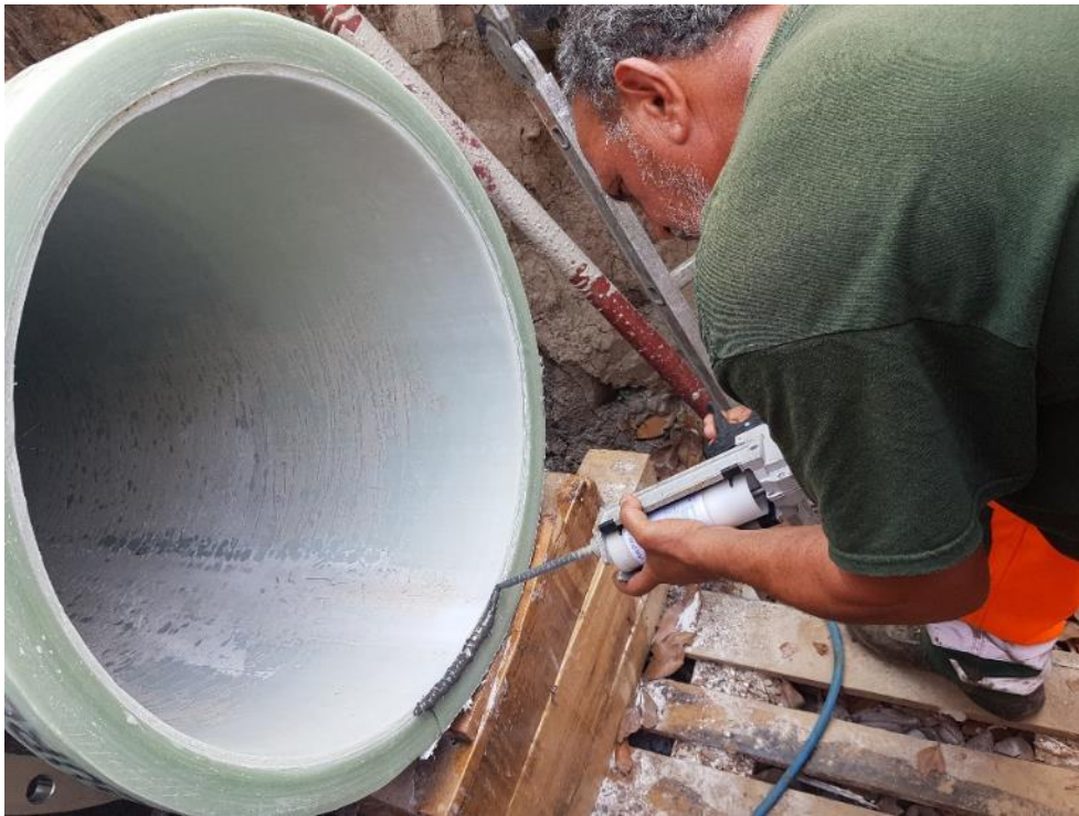
Sealing of the cutting edge
