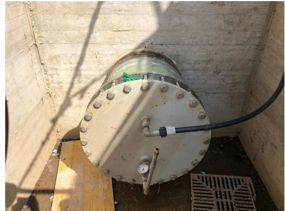
No abudment to counter longitudinal forces
