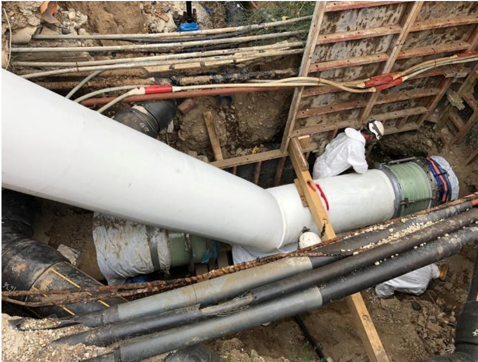
Installation of BlueLiner (Starting point)
