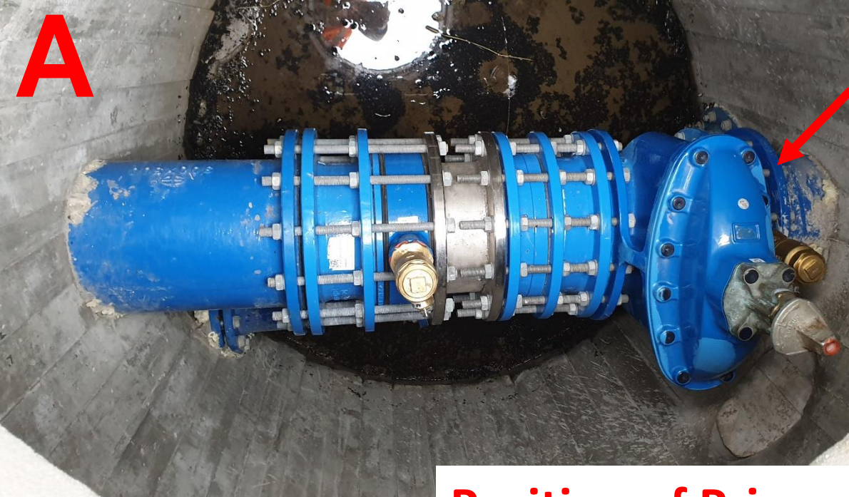
Position of Primus Line Connector
