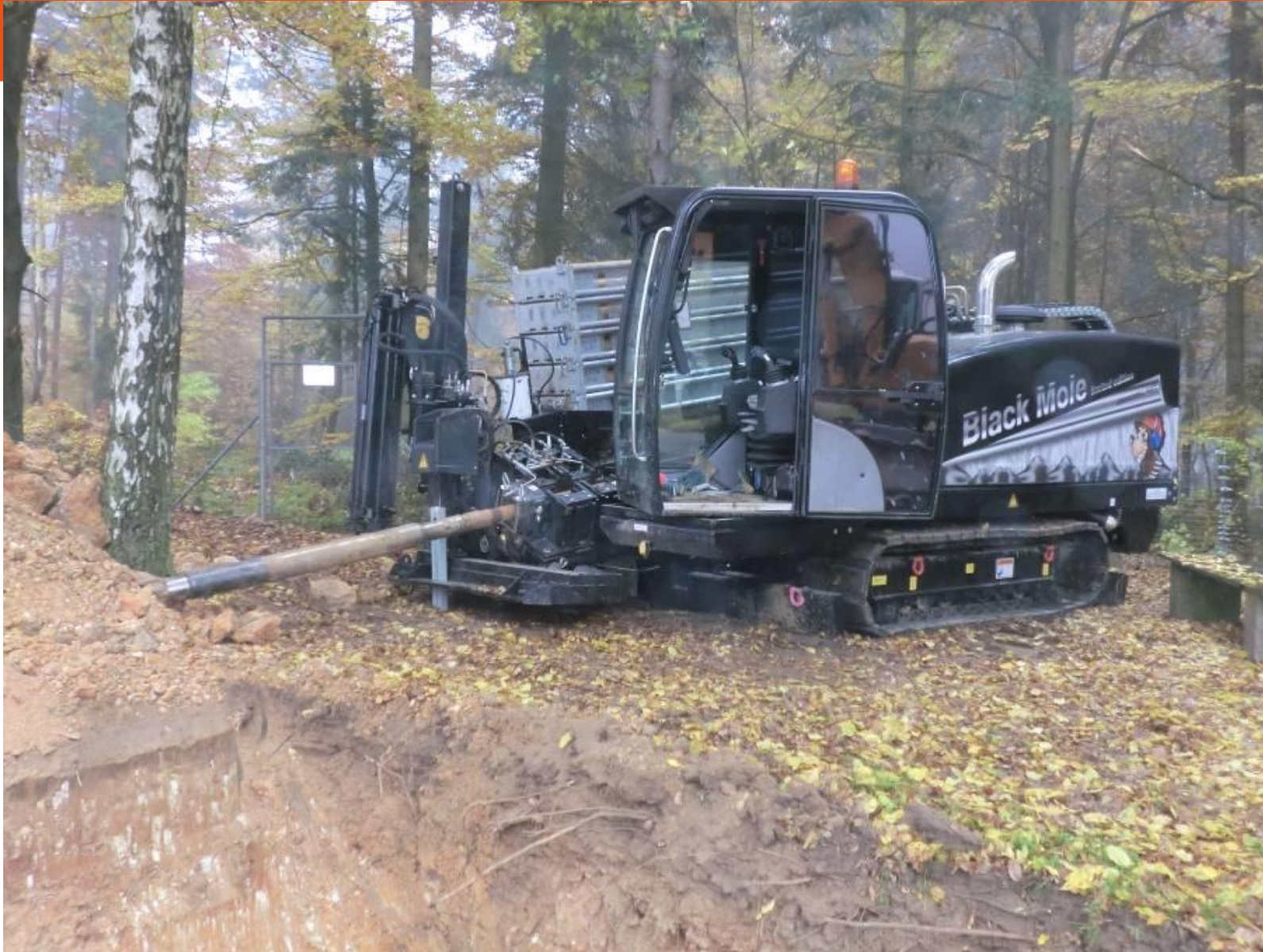
Grundodrill 18 ACS with double rod technology
