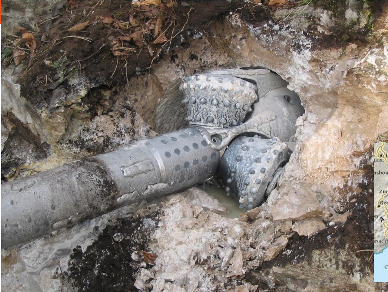
HDD Hole opener in operation in Postojna
